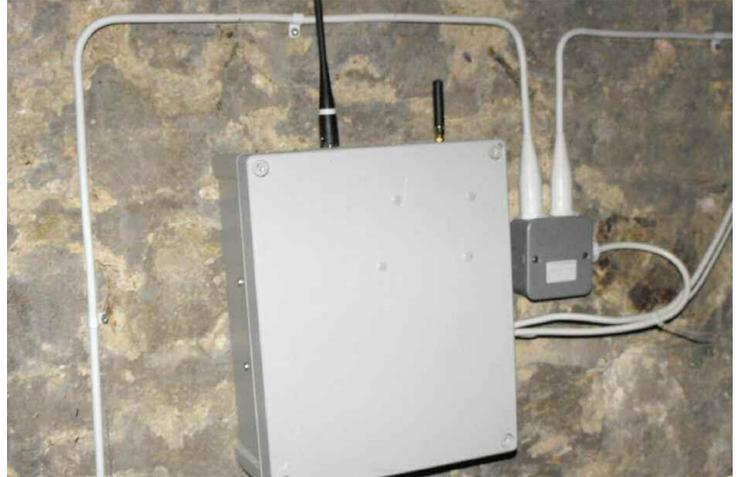
Roof security system panel installed in a church tower
