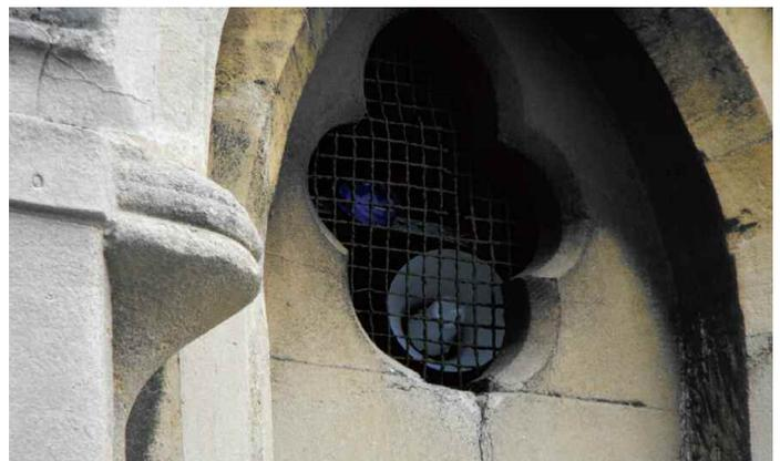
Alarm sounder and blue strobe light installed in a church tower
